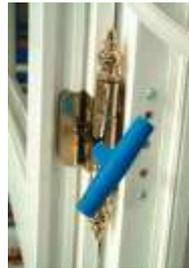
Step 3: Frame grub screw adjustment
