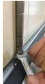
*Step 2: Bifold nut adjustment*
