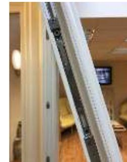
*Fig 2: Exposed Wink Haus gear showing serrated bar to lower section*
