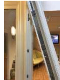
*Fig 1: Shows cover plate in position to be removed for adjustments*
