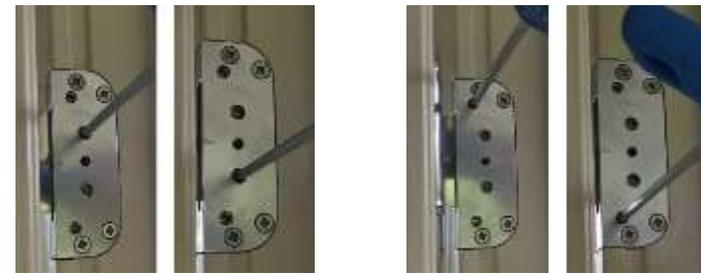
Steps 1 & 2: Inner grub Step 3: Outer grub screw adjustment.
