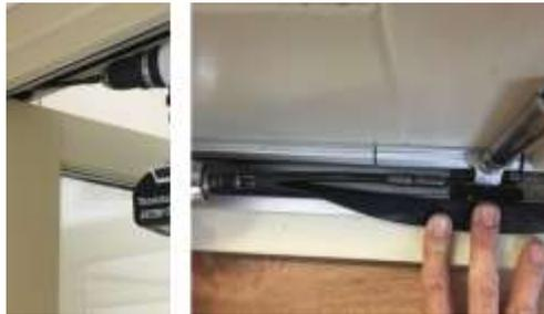
*Step 1: Head & Sill grub screw adjustment*
